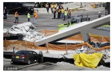
Every element holds clues to what happened – including the cracks in the concrete and stress marks in the metal rods. AP Photo/Wilfredo Lee
