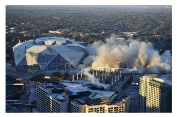
Decommissioning the Dome and preparing it for implosion included removing the seats, video boards and extensive equipment. The impressive implosion lasted for about 15 seconds, with the roof falling in 12 seconds and grandstands coming down in about 3, according to the Georgia World Congress Center Authority, while a five-story industrialstrength curtain was erected to protect the Mercedes-Benz Stadium.
